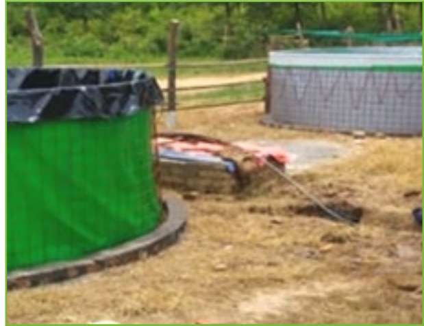
Completed Bio-floc Structure
