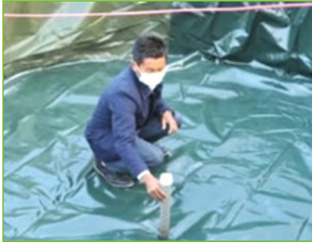
Fixing of UV Stabilized Tarpaulin
