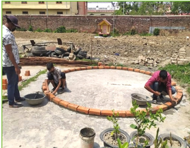
Construction of foundation for installation of Bio-floc
